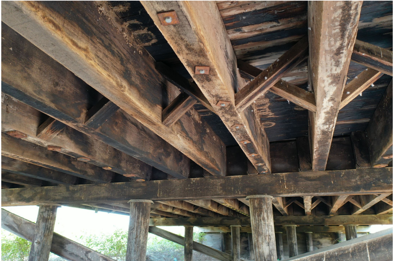
Picture 2 - Repaired Girders
