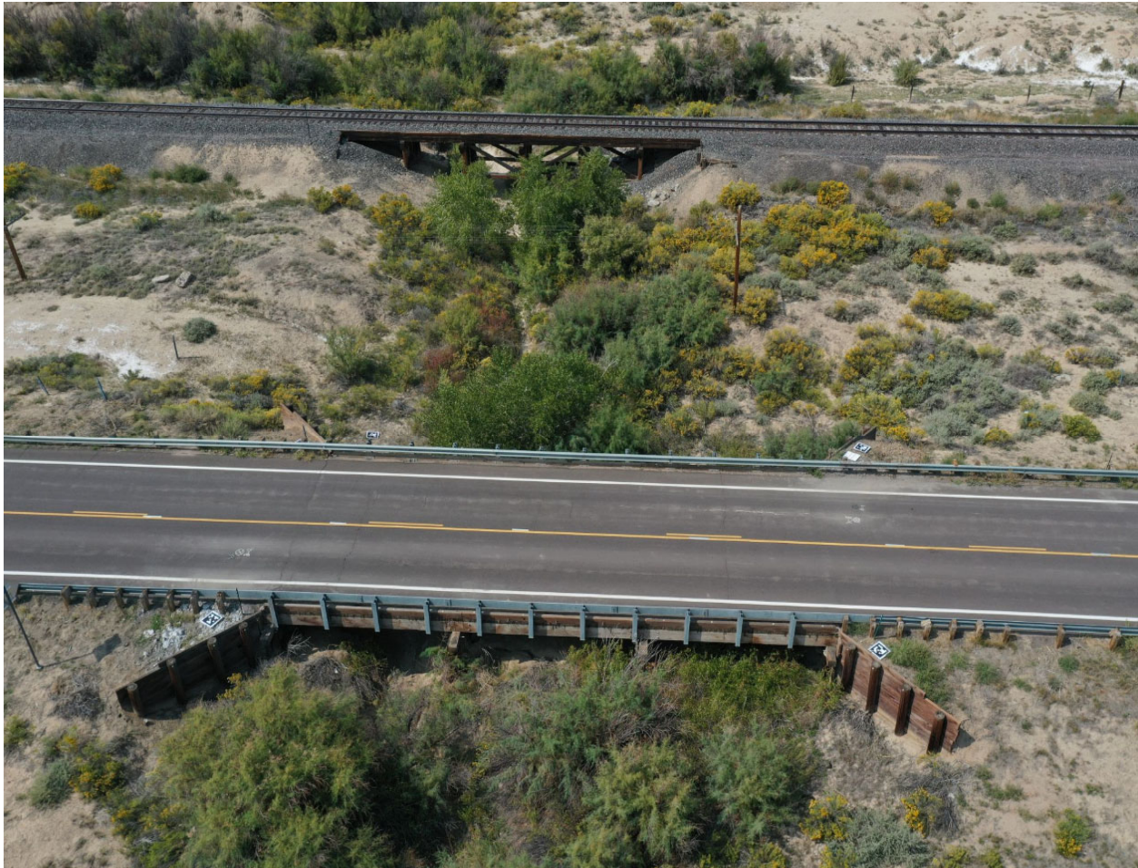
Picture 1 - Bridge O-19-D showing proximity to the railroad bridge upstream
